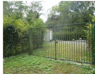
Cesson (77) - Station d'épuration
